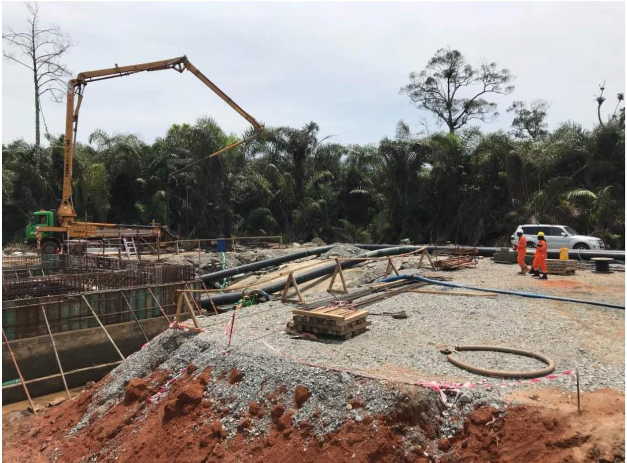
Figure 2: Concrete Casting works ongoing at ENI-Ghana Gas tie-in joint
