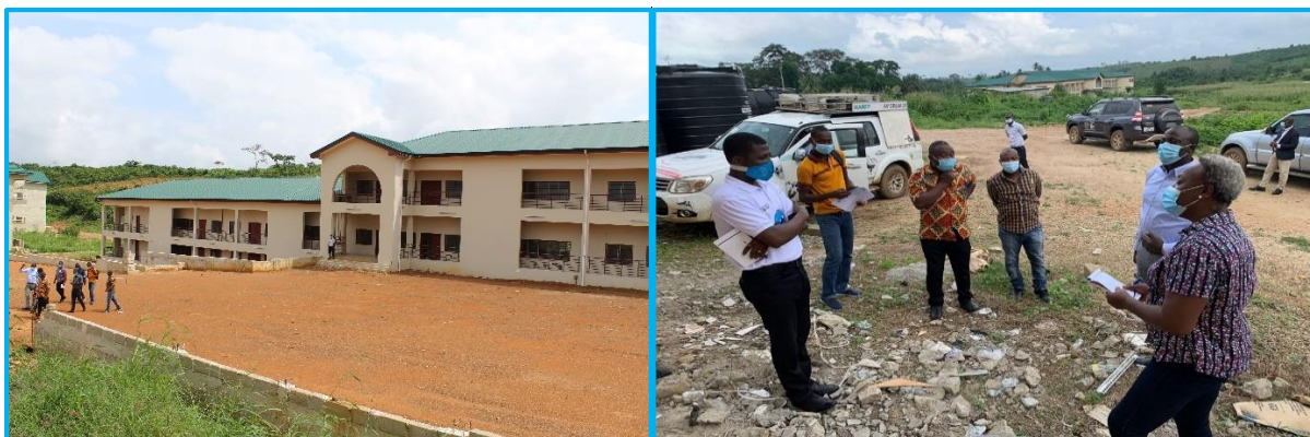
The PIAC team inspected ongoing works at the Anomabo Fisheries College in Cape Coast.
