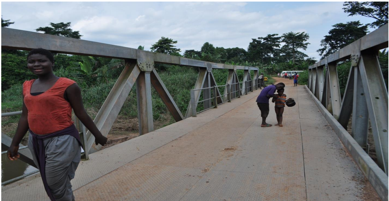
Figure 10: Status of Steel Bridge Over River Dayi
