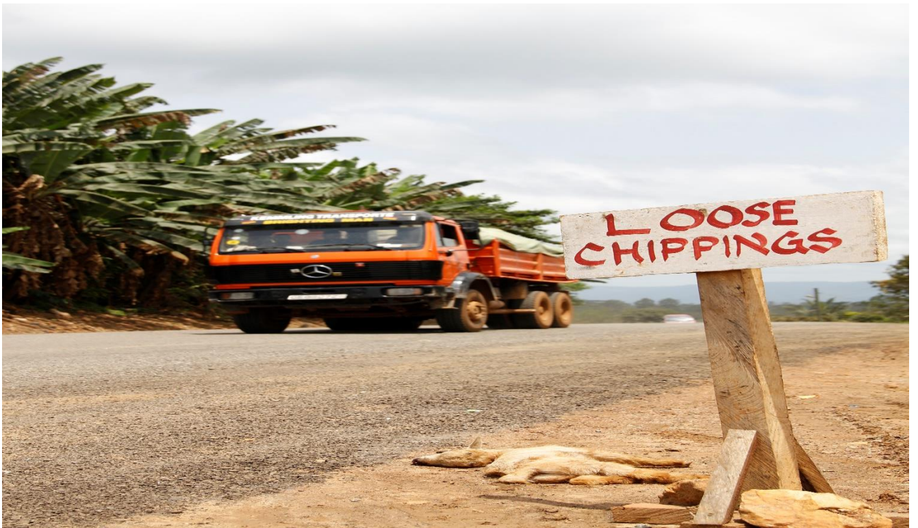
Figure 7: Progress of work on the Anyinam-Kwabeng-Akropong Road
