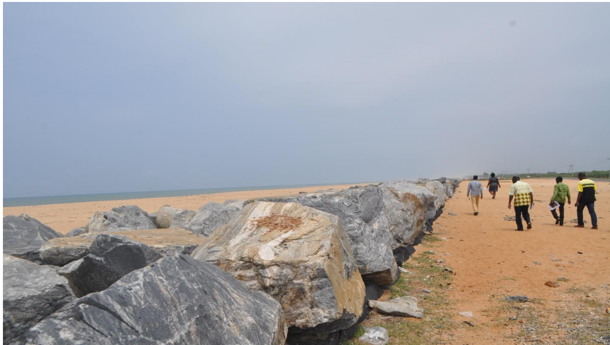
Figure 26: Status of the Sea Defence Works
