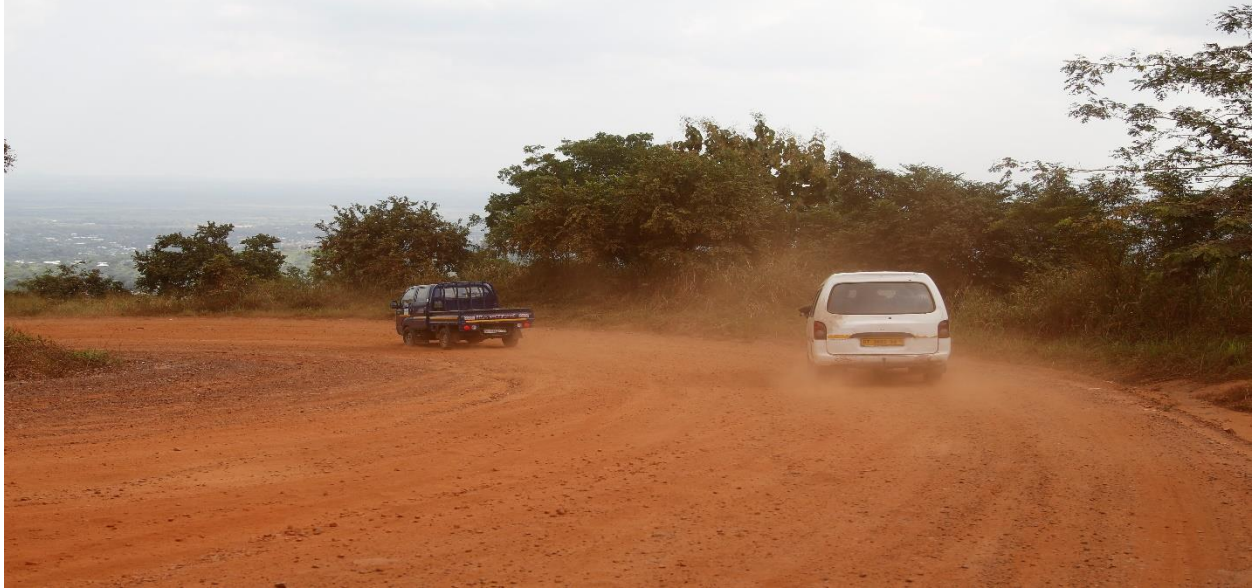
Figure 5: Portion of Odumase Oterkpolu Road under construction
