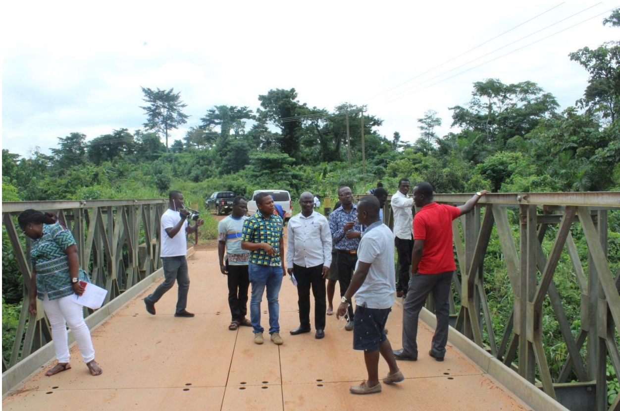
Figure 3: Steel Bridge Over River Ponpon at Ponponso, East Akim
