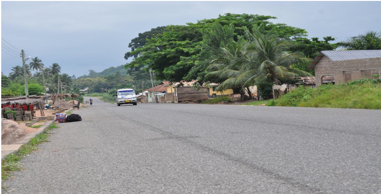
Figure 8: State of a section of the Ho - Adidome Road
