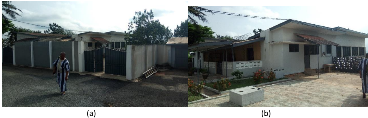
Figure 22: Headmistress' Bungalow (a) View from Outside (b) View from Inside
