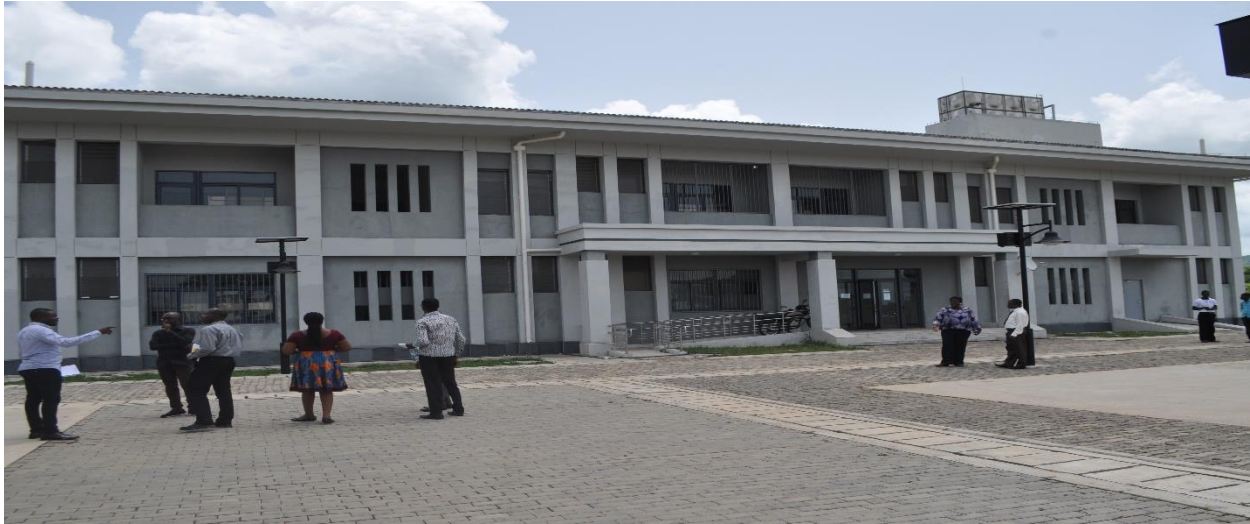
Figure 25: The 2-Storey Hostel Block at UHAS
