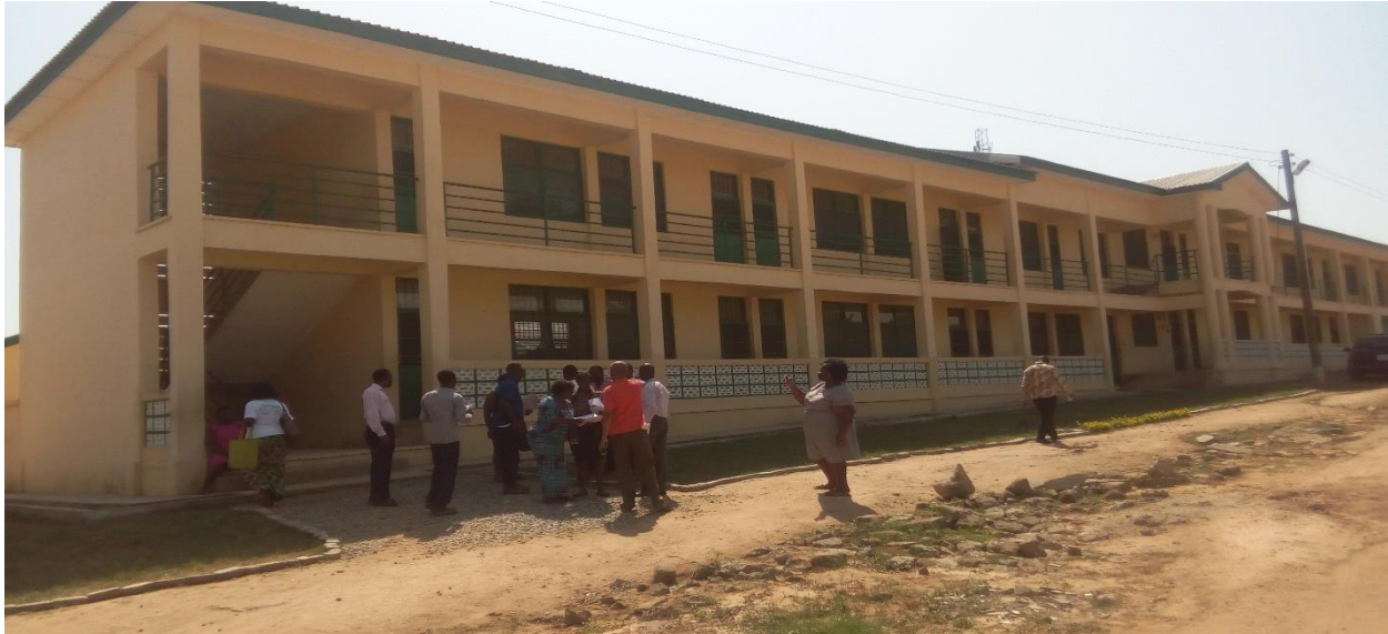
Figure 31: State of 2-storey Dormitory Block at Odorgonno SHS
