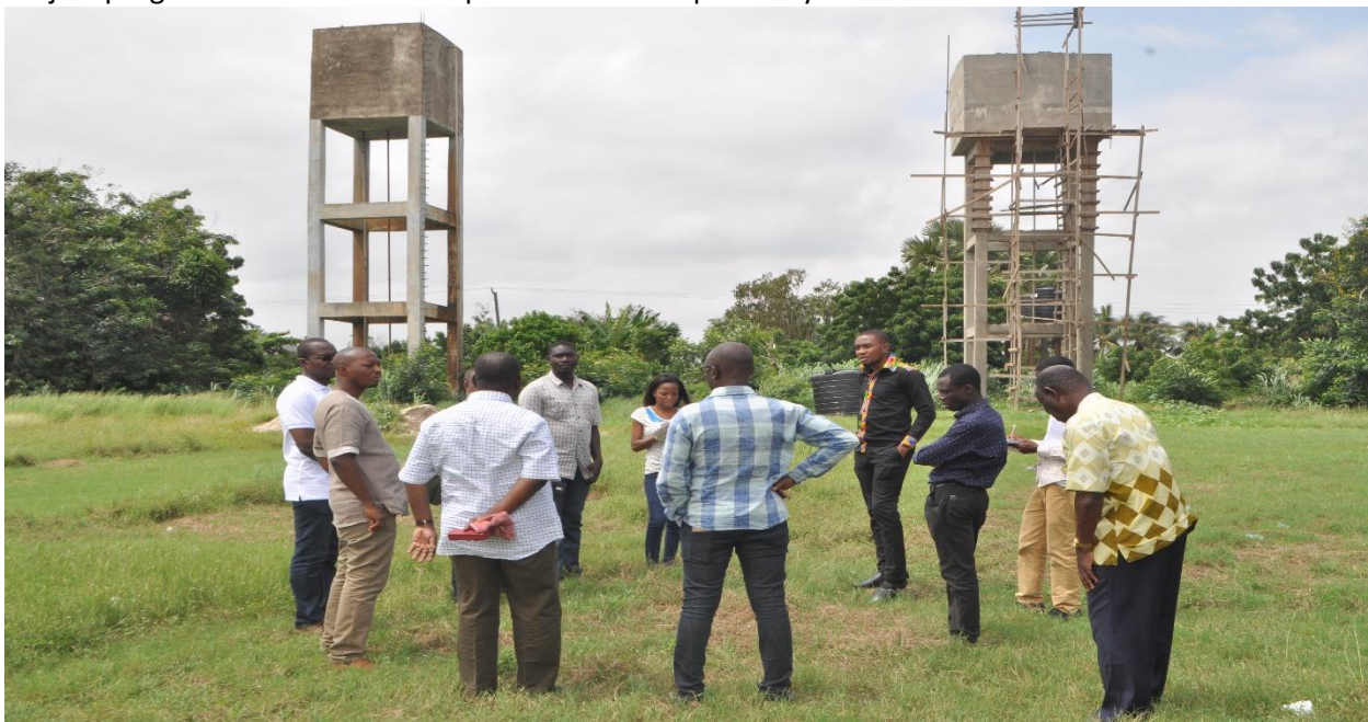
Figure 27: State of Water Supply Projects
