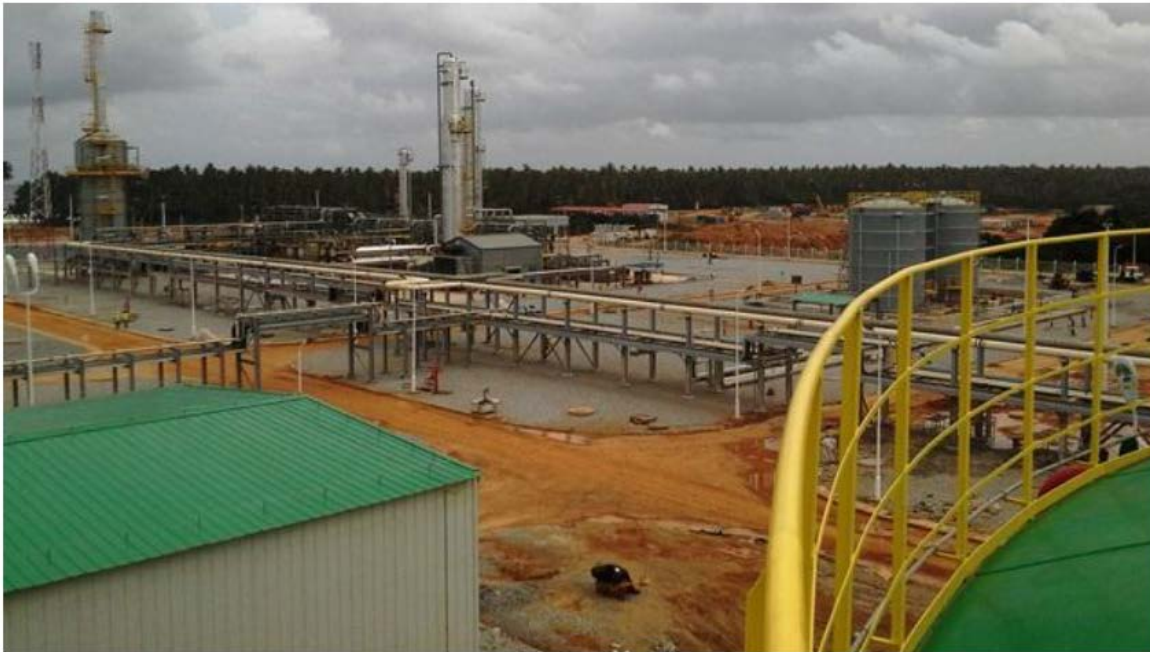
FIGURE 1: PICTURE OF THE GAS PROCESSING PLANT UNDER CONSTRUCTION
