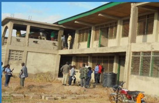
Two-storey dormitory facility at Zebilla SHTS
