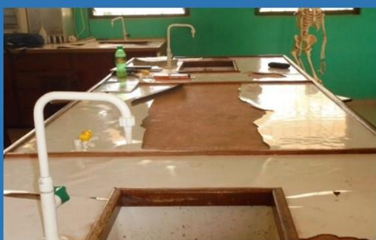
State of rehabilitated Science laboratory at St Francis of Assisi SHS
