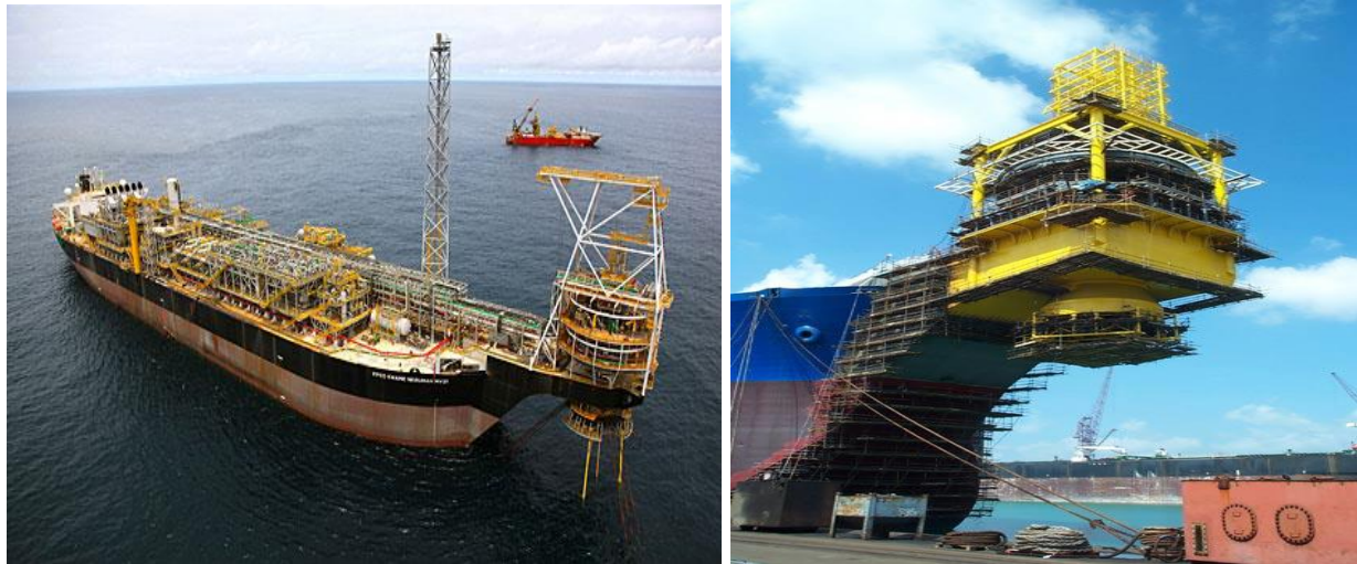
FIGURE 1: PICTURE OF FPSO KWAME NKURUMAH (L) AND UNDERSIDE OF AN EXTERNAL TURRET(R)
