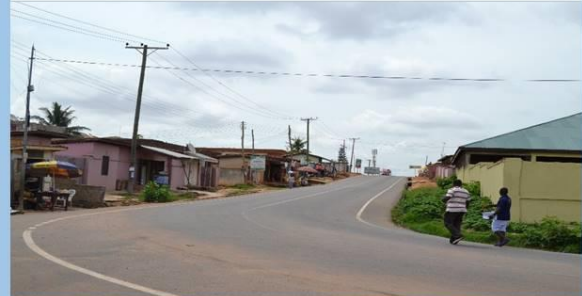
PIAC-IFEJ team inspects Sepe-Dote Road
