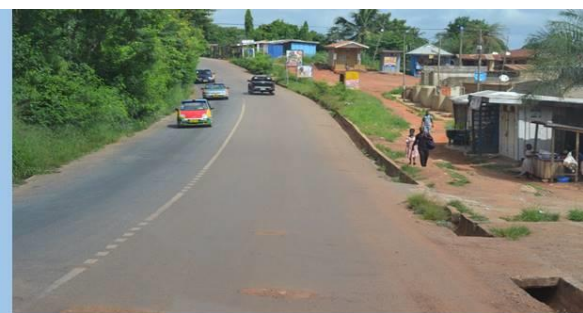
State of Bremanng UGC road
