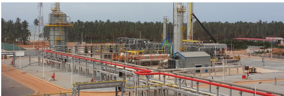
Figure 14: Atuabo Gas Processing Plant
