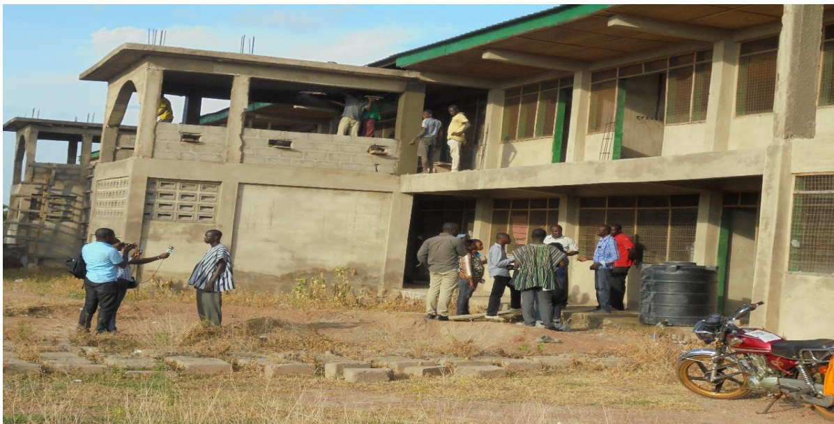
Figure 1: Progress of work on the two-storey dormitory facility at Zebilla SHTS
