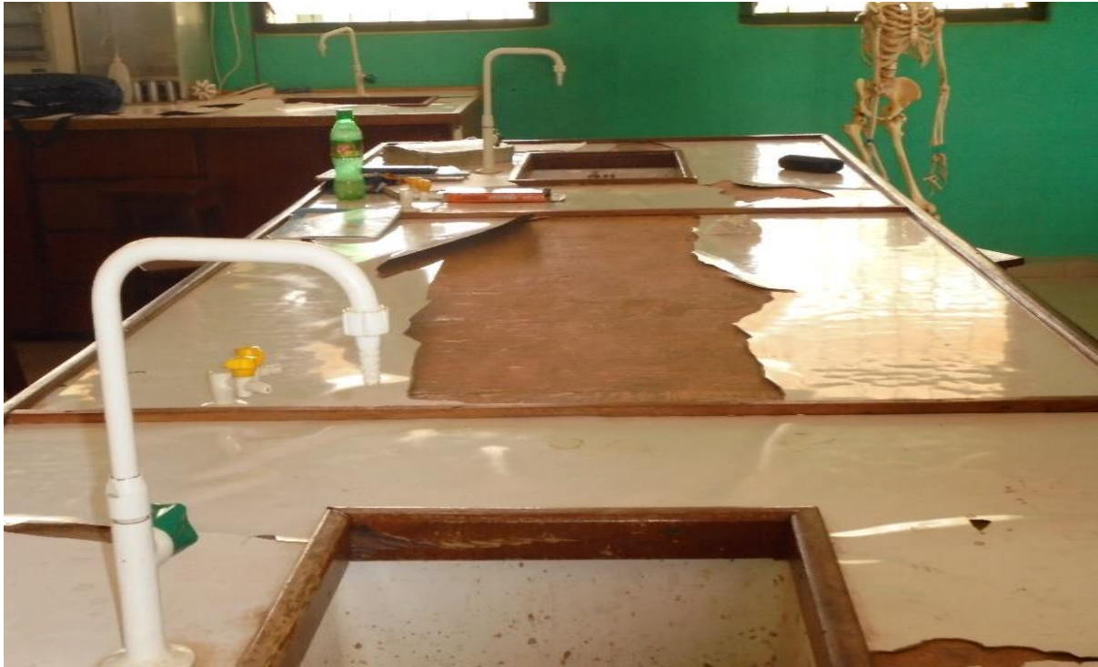
Figure 3: State of facilities at the rehabilitated lab at St. Francis SHS
