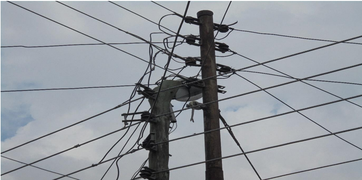
Figure 6: New cables fixed alongside old cables at Bagabaga College
